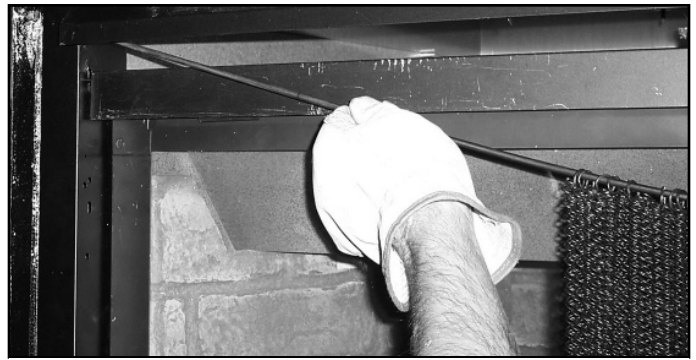
Figure 14.15 Insert Rod Into Side Columns
